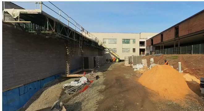
Between Gym & Existing Covered Patio
