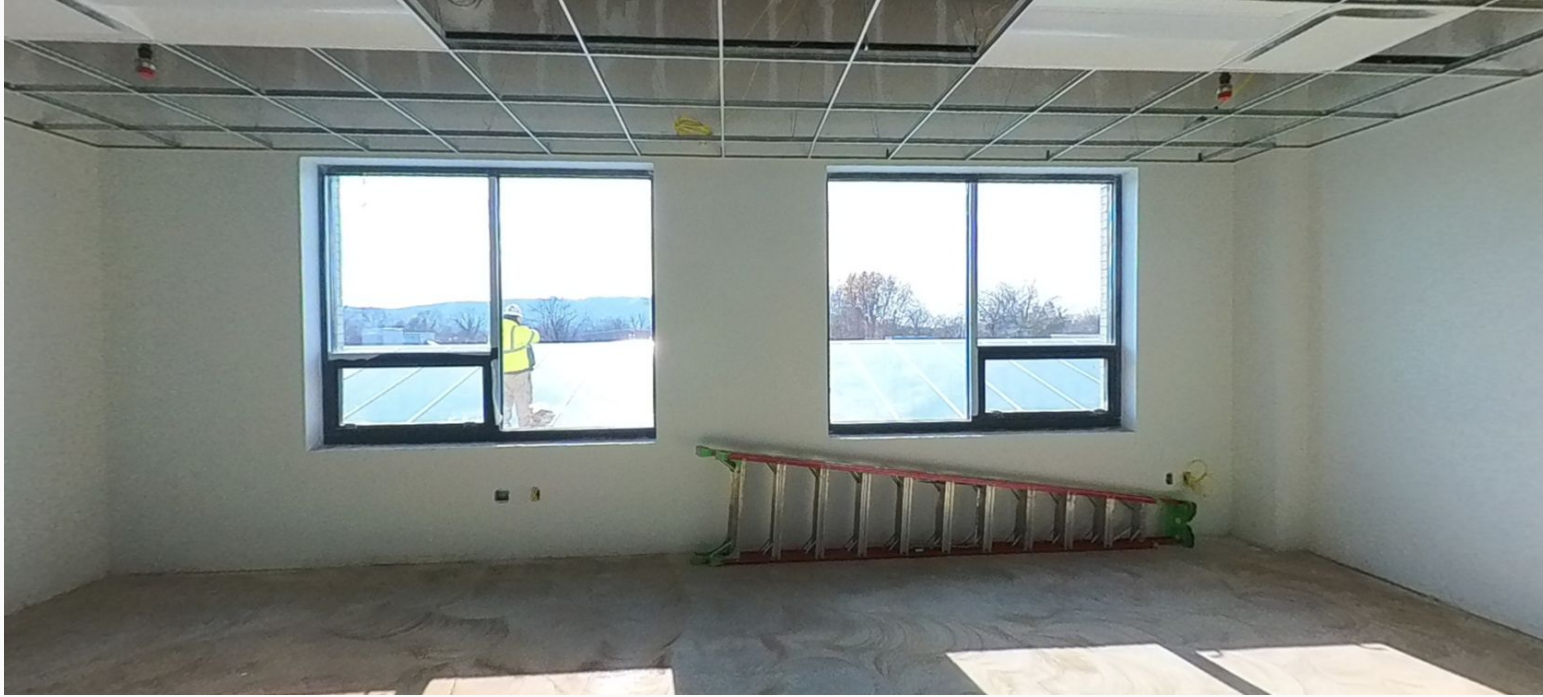
Typical Classroom - windows, ceiling grid, drywall
