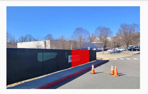
A gate <u>may</u> be installed in the construction fence beside the bus loop (highlighted in red on the picture below) to allow trucks to enter the site through this location. Nielsen will only schedule deliveries between the hours of 9AM and 2PM, and they will also be employing a 'crossing guard' to ensure that children can walk safely to the Boys & Girls Club, and to ensure no issues with traffic when trucks are present.
